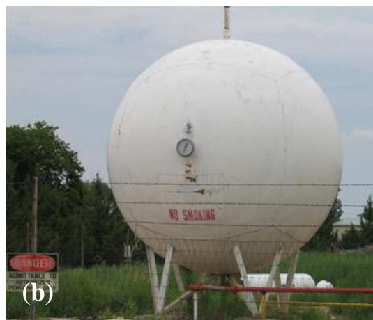
Figure 1: Pressure vessels: (a) cylindrical tank, (b) spherical tanks.
