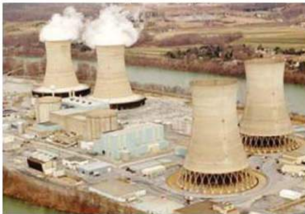
Nuclear Power Station
