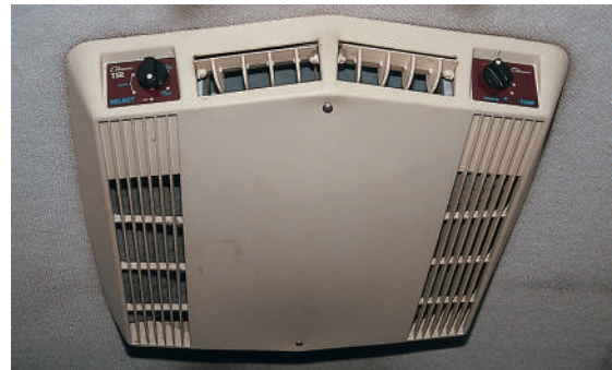
Figure 47-8 Part of the control circuit is located inside, under the front cover. Photo by Bill Johnson
