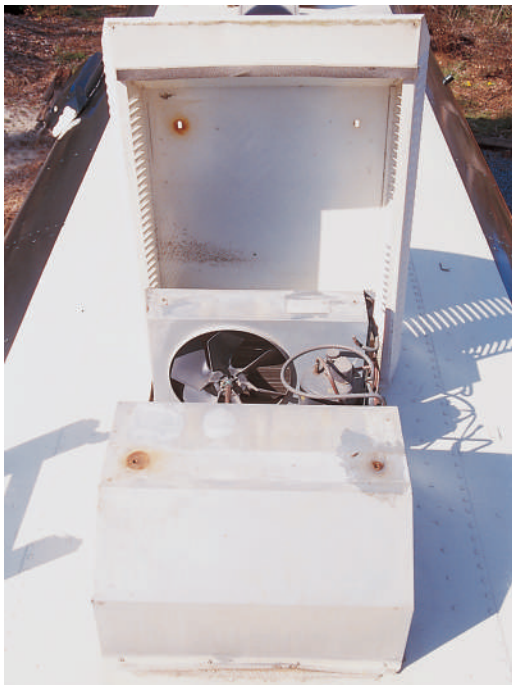
Figure 47-7 The case lifts off the roof-mount unit. Photo by Bill Johnson
