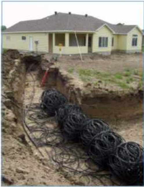
Figure 4. Horizontal "slinky" system installation (before)
