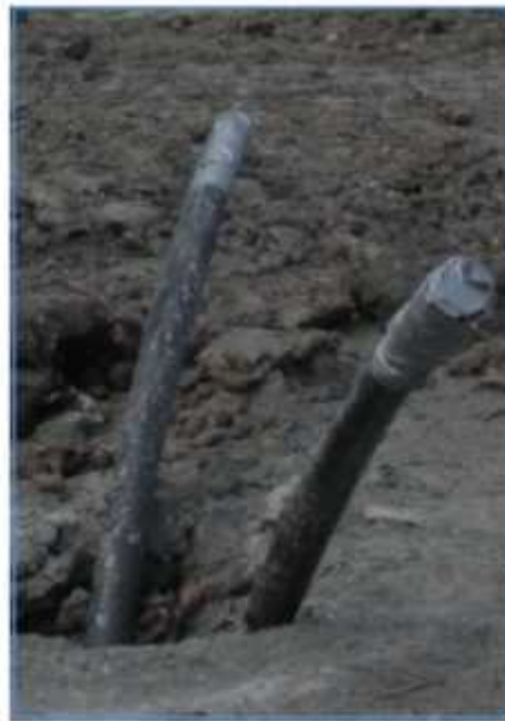
Figure 7. Installed vertical ground loop
