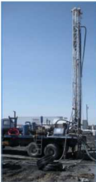
Figure 6. Drill rig installing vertical ground loop
