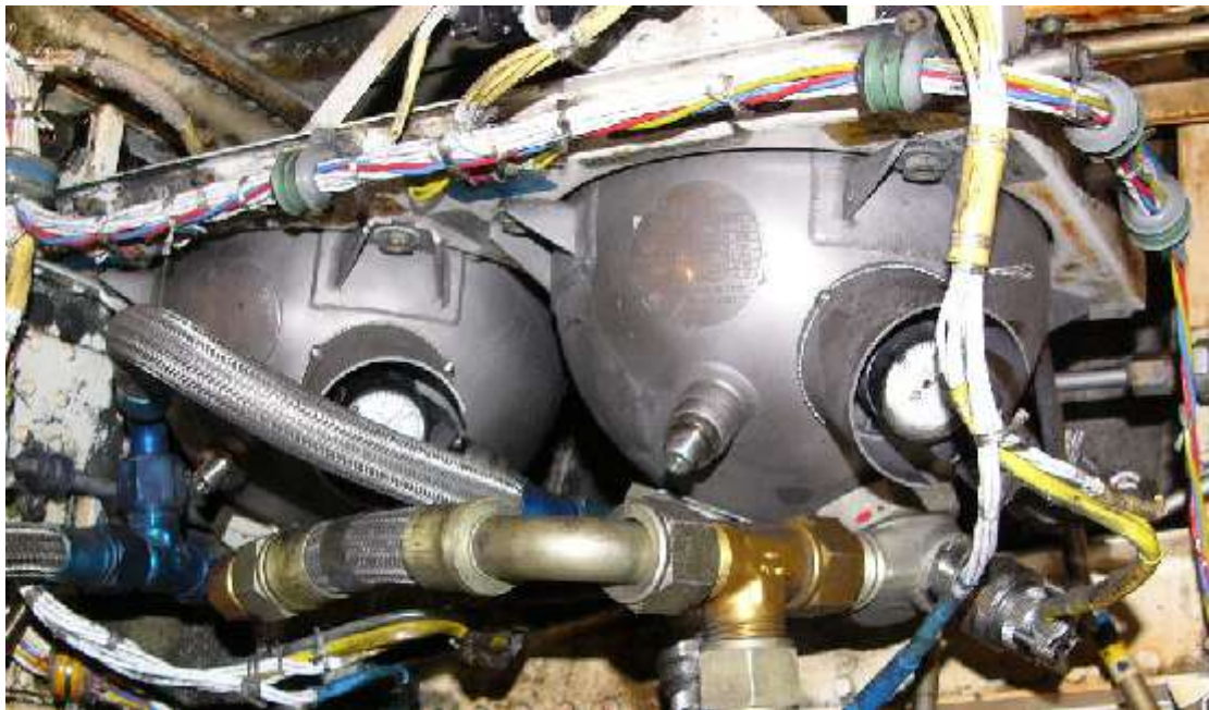
Fire Safety System in Boeing 737
